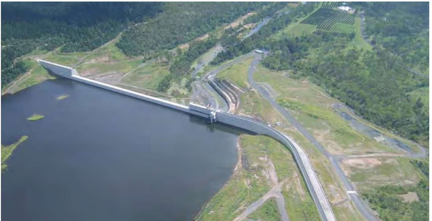
Construction of SunWater's 300,000 megalitre Paradise Dam and the 20,000 megalitre Kirar Weir in Bundaberg, Queensland, has provided local growers with another option for sourcing water. Paradise Dam has reached record levels of 45 per cent capacity and Kirar Weir was almost full, said SunWater's Garry Grant. The water supply is to be used for agricultural, industrial and urban sectors.
