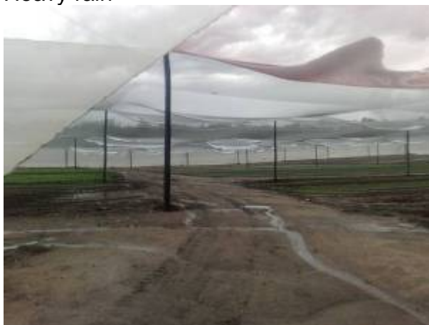
[Image 20 –heavy rain accumulation on top of a supported hail net]
