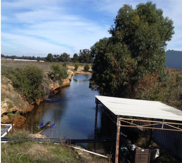
The ditch is fed by three bore pumps positioned across the farm. These are each 7.5 kW pumps running at about 60% of their maximum. This provides a good opportunity for Ivankovich Farms to switch over to solar bore pumps, or to add VSD drives to reduce the power draw of these pumps and save energy.
