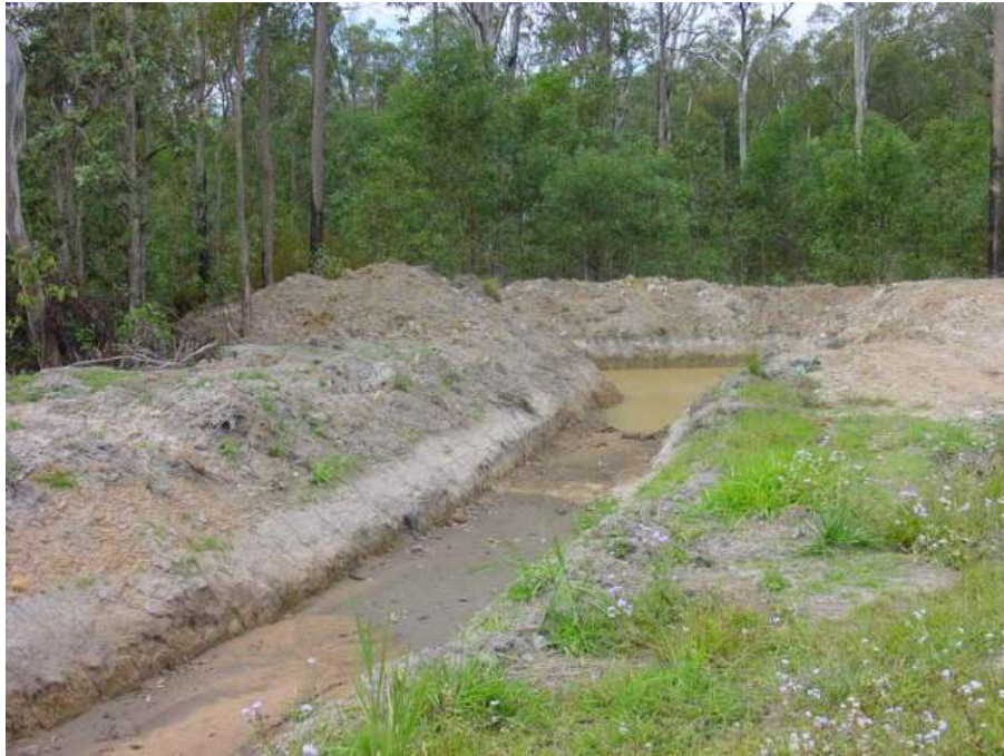
Figure 2: Example of a silt trap on a pineapple farm, SE Qld.
