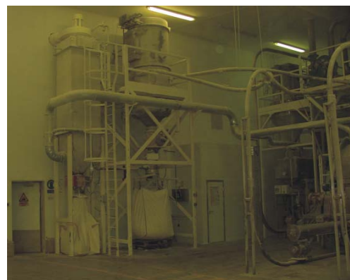
The Mills are in a separate controlled-atmosphere room. Product can be dropped into a silo for storage or into a transporter for immediate delivery.
