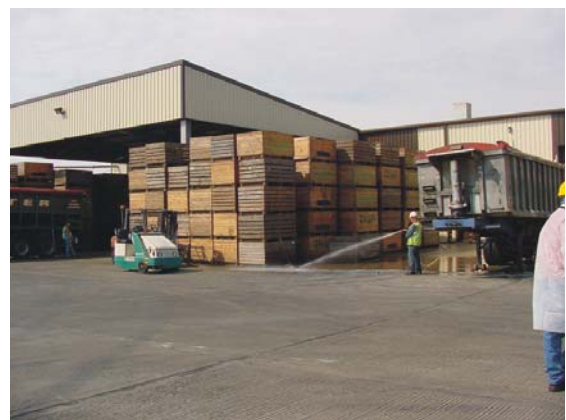
The delivery and storage area which is about to be upgraded.
