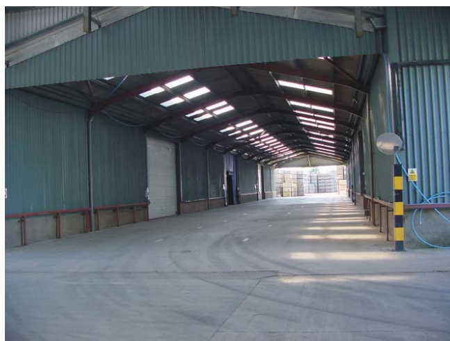
Burrelton’s large storage area – there are 6 storage rooms branching off of this central loading bay.
