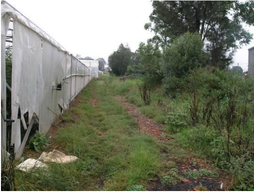
Figure 15. Side fence 'Before'
