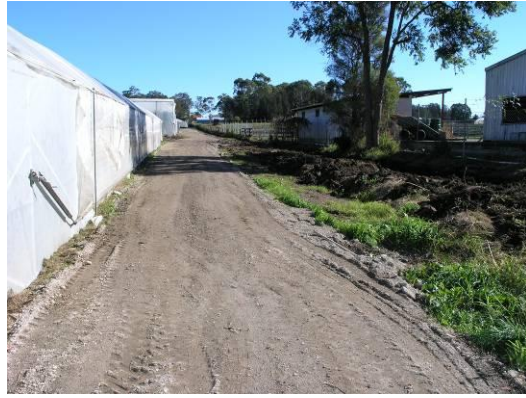
Figure 16. Side fence 'After'
