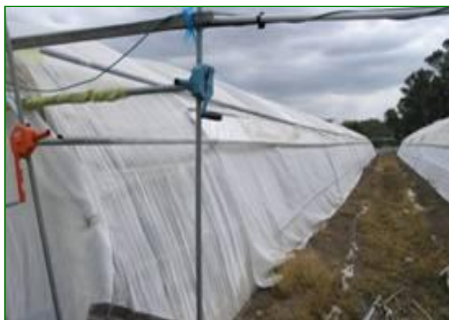
Figure 14. Tunnel greenhouse in Rossmore with roll up sides protected by whitefly grade insect screening
