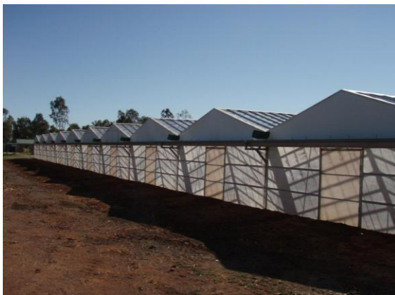
Figure 10 Low technology greenhouses on Property 1 on Northern Adelaide plains, glass (left) and plastic (right).
