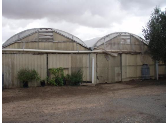
Figure 15 Low technology plastic greenhouse on Property 2 on Northern Adelaide plains
