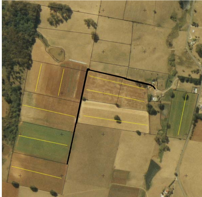
Fig 9. Existing layout showing access road (black) and direction of operations (yellow) in each paddock.
