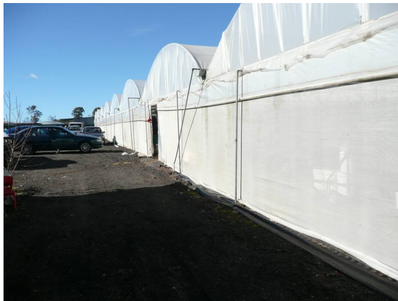
Figure 10. Greenhouse 4, a medium technology greenhouse showing detail of roll up side wall vent with insect screen installed.
