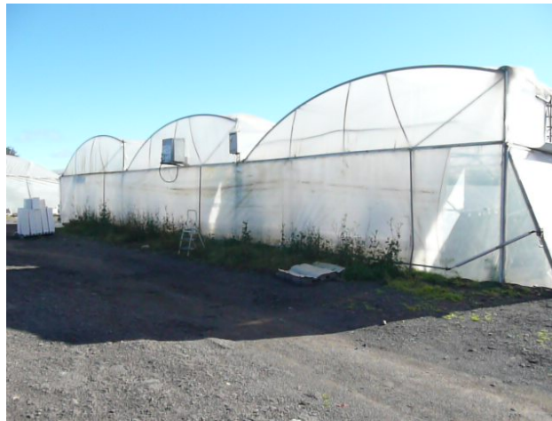
Figure 12. Multi-span greenhouse with sidewall rolling vent and rolling roof vent (unscreened).
