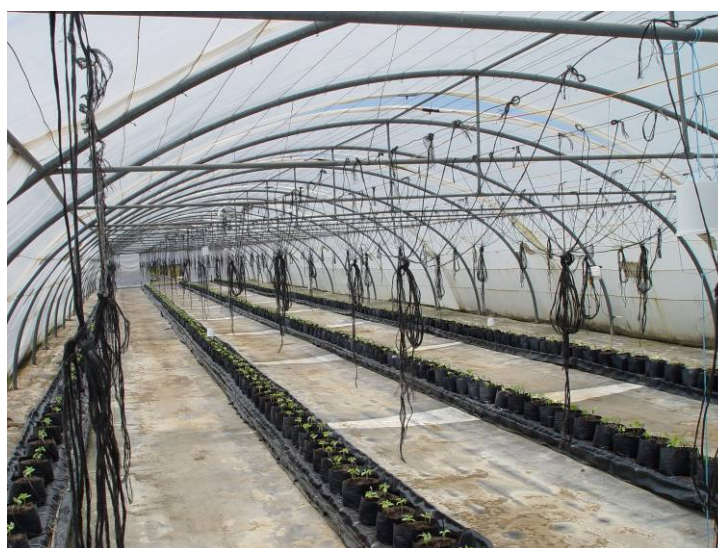
Figure 8. Greenhouse 3, a low technology tunnel house showing detail of a rolling roof vent.
