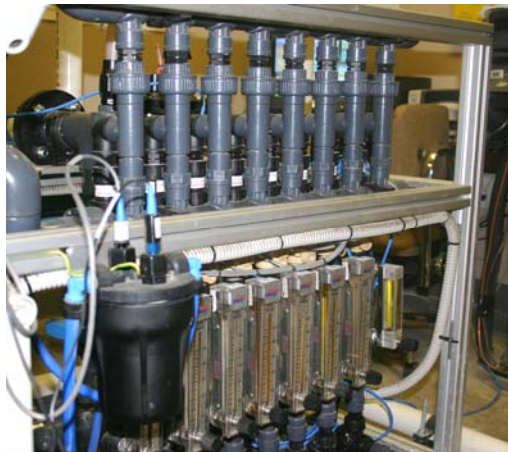
Nutrient management and irrigation of the greenhouses is all controlled by a 'turn key' computer controlled system.
