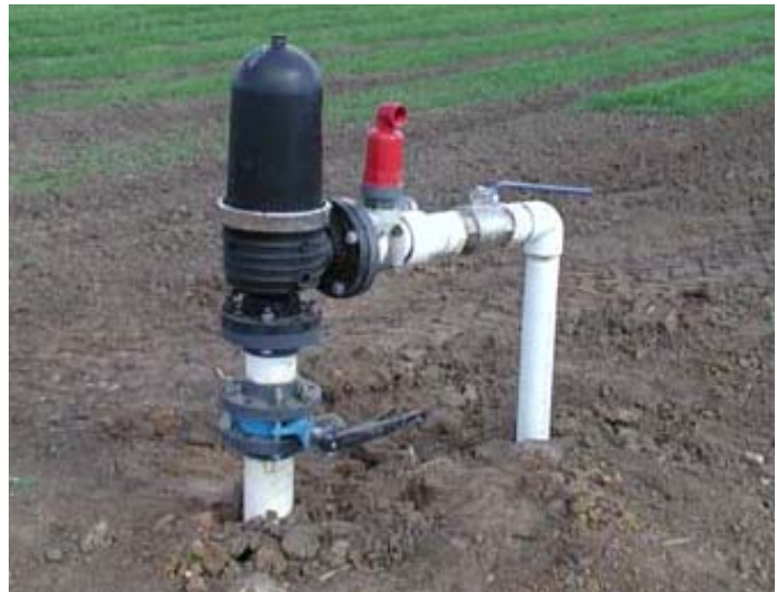
Fig. 7: New irrigation sub-main.
