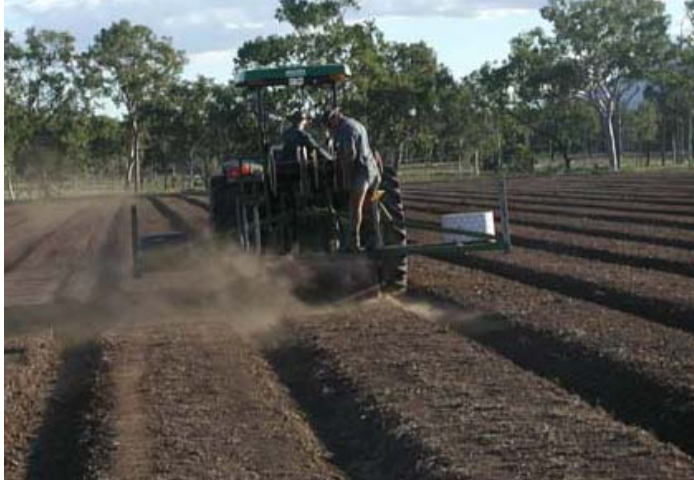
Fig. 9: Installation of heavy duty drip tube.
