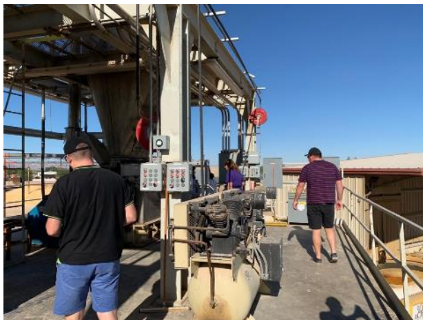
El Toro feedlot plant mixing station.
