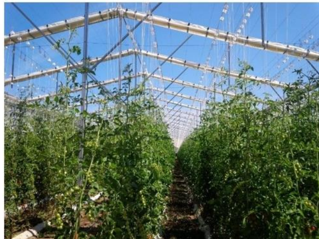
Figure 10. Examples of retractable roof structures with peaked roofs. There are also models with flat roofs used in overseas regions where rainfall is low. A commercial retractable roof structure in Bundaberg was setup in 2015. Four extreme weather events (storms with intense wind and rainfall) between 2015 and 2017 demonstrated the level of protection that these structures can provide to vegetable crops (tomatoes and capsicums). On sunny days, the roof can be opened totally or partially to modify solar radiation, soil and crop temperatures, and air relative humidity. Similar structures have been operating in warm climates such as Florida, USA, Mexico, South Africa and Turkey (Image source: (Images source: DAF and < https://www.cravo.com >).
