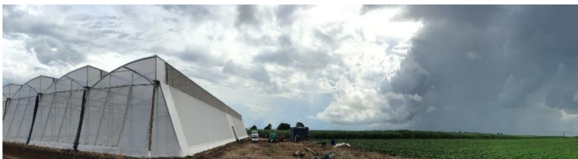
Figure 9. Examples of high passively ventilated greenhouses with roof vents used in the tropics (Image source: DAF).
