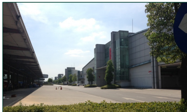
SHANGHAI: vast site – massive investment
