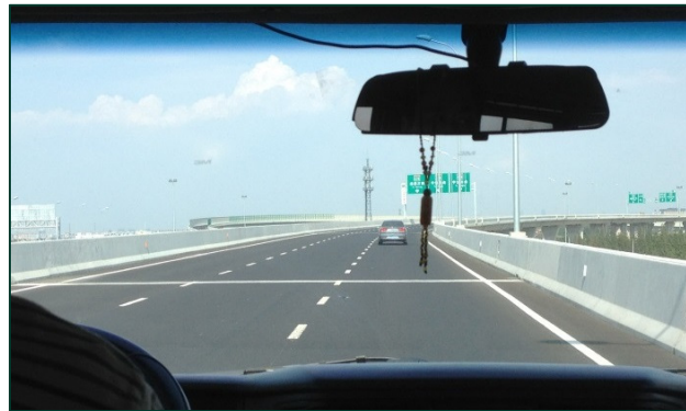
SHANGHAI: dedicated motorway spur to facilitate transport
