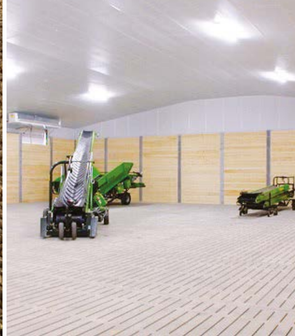
Figure 5. The best bulk storage facilities use fully vented floors. Image: Wolf Systems Canada.
