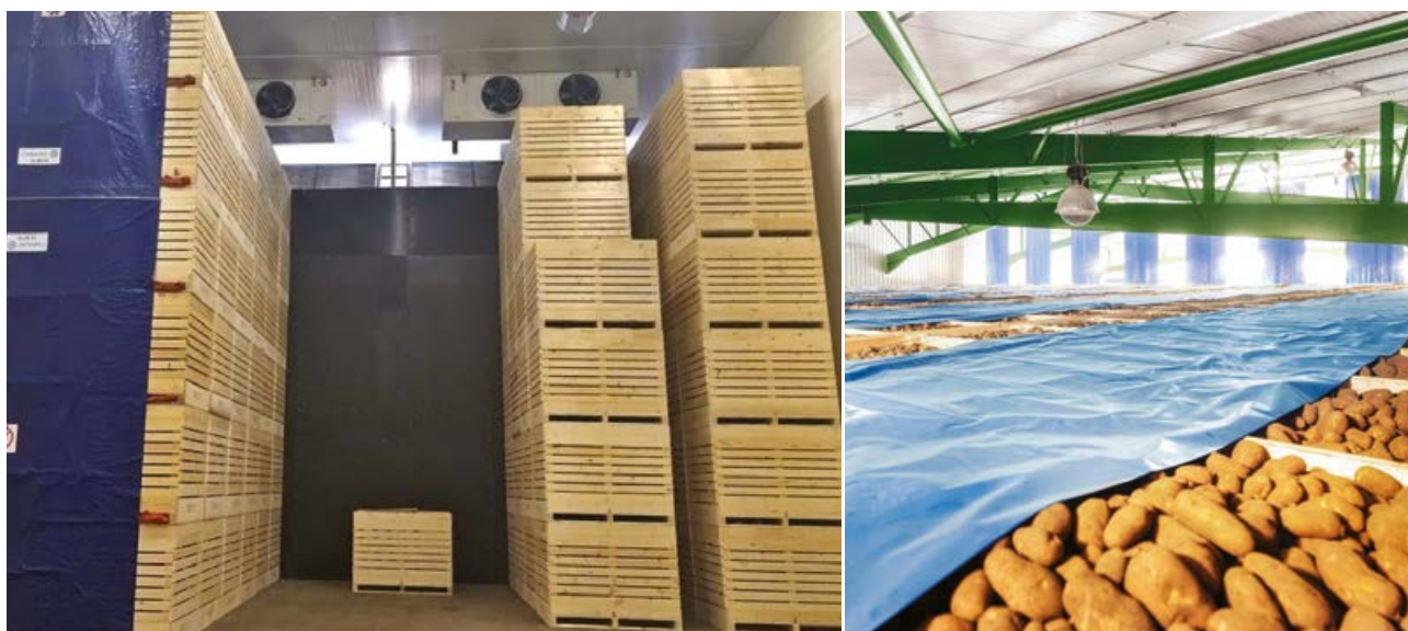
Figure 8. The Omnivent suction (forced air) system actively pulls air through bins rather than blowing it over the top, providing rapid drying, curing and cooling. Images: Omnivent.
